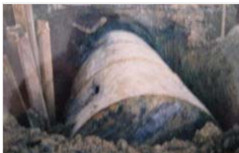
Leaking underground storage tanks are one source of hazardous substance liability
